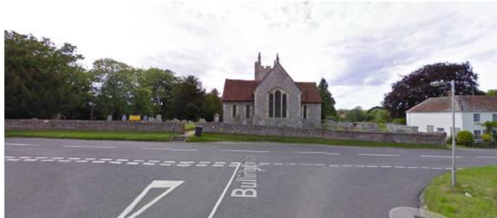
All Saints Church, surrounded by brick and flint retaining wall Image taken from Google Street View
